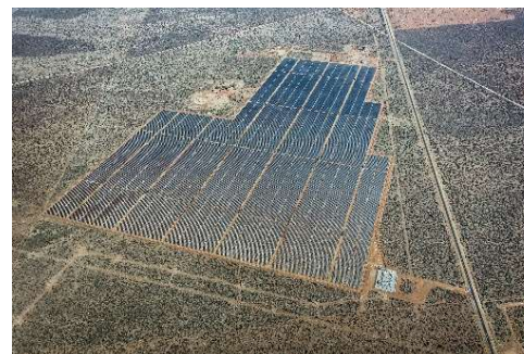
Katu (South Africa) Solar 82MW
